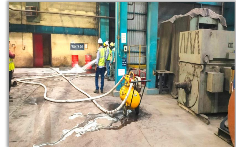
MOT fire fighting Mock Drill at Barmer
